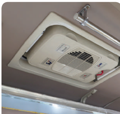
Emergency Exit With Roof Ventilator
